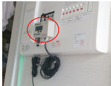
Figure 2. Measuring device installed at the home distribution switchboard.
